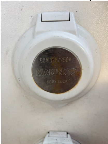
Top Plug – Use with 50amp cord when 50amp 250V is available.
