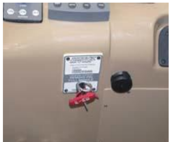
Engine Room Fire Extinguisher emergency control is located on the lower helm. Pull pin and then pull handle to activate.
