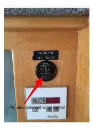
Now gas will be allowed flow to the stovetop. Depress stovetop knob for desired burner and turn to desired flame setting. Hold in the burner knob in the down position for 3 seconds before releasing to allow thermocouple to remain in the open position. Happy Cooking!
