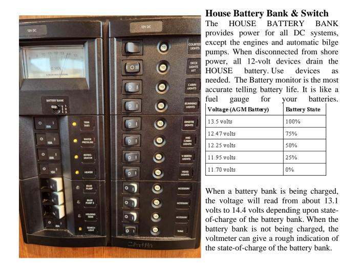
All batteries are charged by the engine ALTERNATOR while underway, and by the BATTERY CHARGER when connected to shore power. The Solar Panel will also charge the Engine and House batteries automatically.
