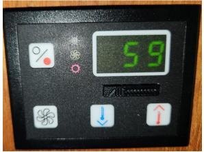
This system uses AC power to provide both heating and air conditioning. Press the up and down buttons to set the temperature, fan button changes fan strength. NOTE: fan speed numbers; higher # = slower fan
