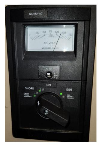
At the ELECTRICAL PANEL, flip the two AC MAIN breakers on. Green lights on the panel should come on. Then rotate the switch below the AC breaker panel to the SHORE setting. Turn on desired outlets on panel.
