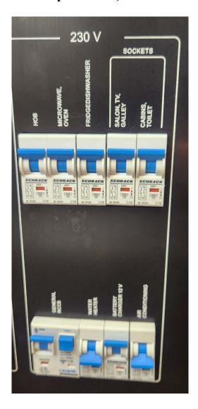
SHORE POWER supports all AC equipment and receptacles on board, as well as the battery chargers.
