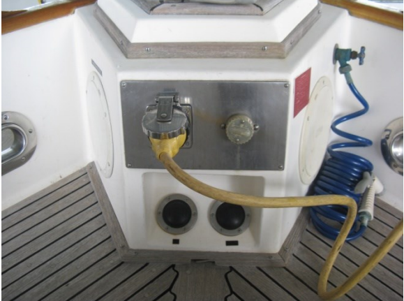
FORWARD SHORE POWER CONNECTION
