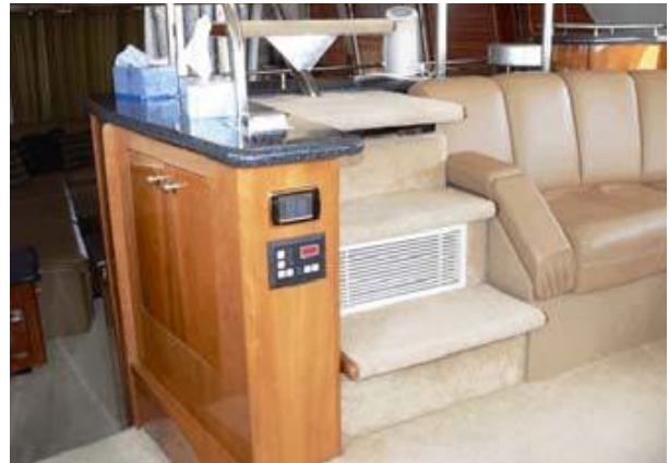
Steps to the flybridge with the AC power panel cabinet at their base.
