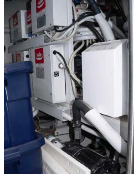
[above] Starboard lazarette: Air conditioning controls with compressors behind and seawater pump below. Engine spare parts/supplies in the boxes. The starboard lazarette also holds stern thruster batteries & misc. supplies.
