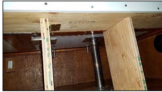
13. View from below after attached.
