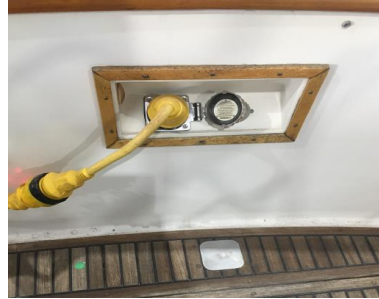
Aft power connection
