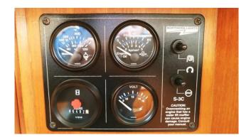
After generator is running, turn your AC distribution switch to generator. Then turn on AC systems as you would on shore power one system at a time.
