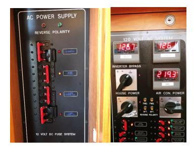
At this point you can turn on appropriate breakers for battery chargers, refrigeration, water heater, and remember the inverter input and output need to be on for charging. Watch your volt meter for load. If the load exceeds 50 amps, you will pop your dock breaker. If this occurs, wait to turn on one of your systems (i.e. water heater) until your use of volts drop.
