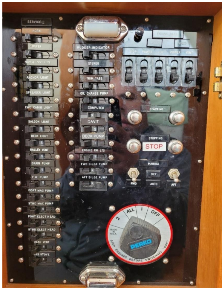
12 Volt system, engine start, and battery selector
