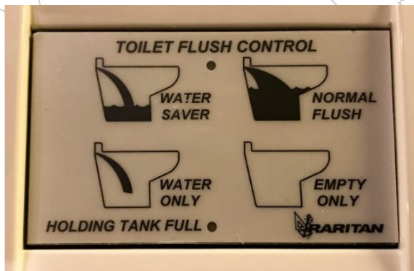
Figure 5 - Toilet Flush Control
